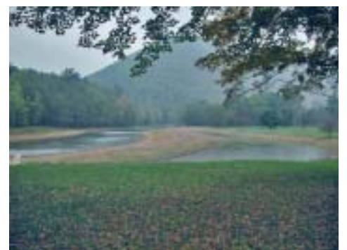
Left: In 2005 vegetation is taking hold. The constructed oxbow is working as designed to catch sediment during times of high flow.
