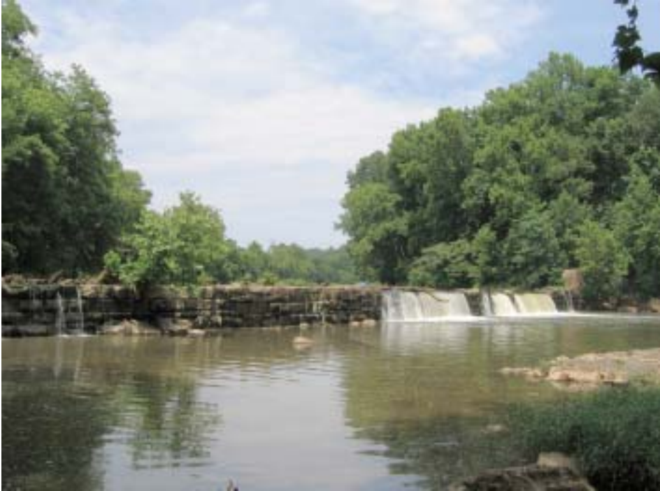
Removing part of the long-neglected Woolen Mills Dam would reopen over 20 miles of the Rivanna River to migratory fish. Photo courtesy of Jason Halbert.
